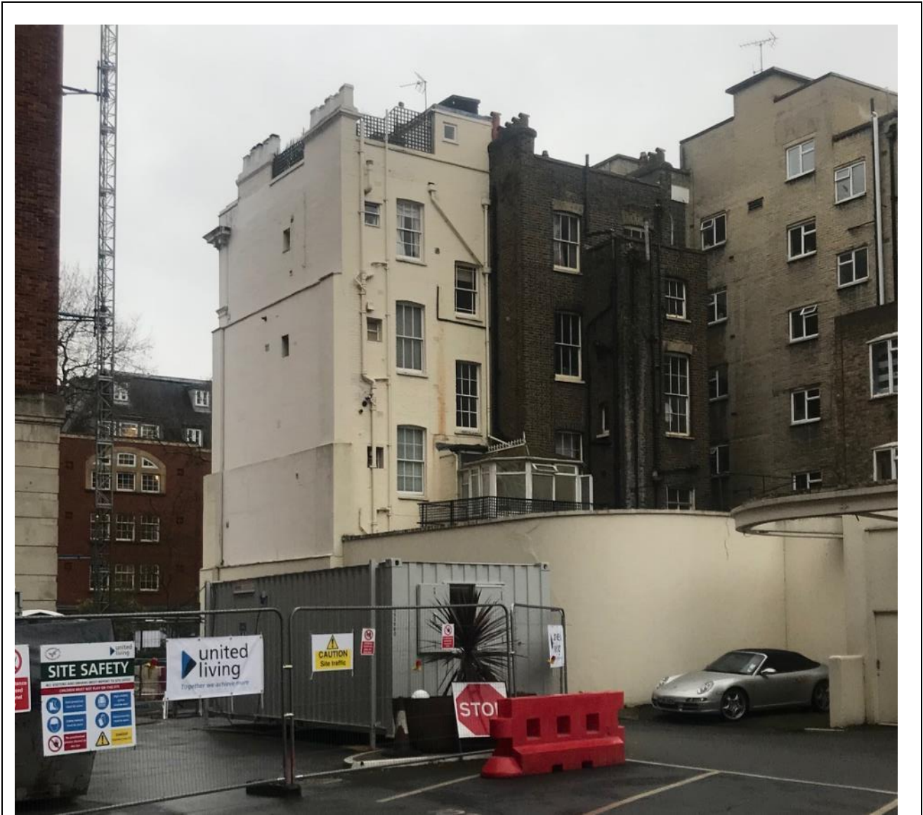
View from Dolphin Square Car Park
